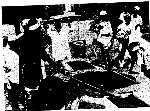
Figure 5.9 A well with a headwall and rollers in Nigeria. The arrangement prevents surface water running into the well and also prevents Guinea worm transmission at the well. (Photo: R Feachem)
