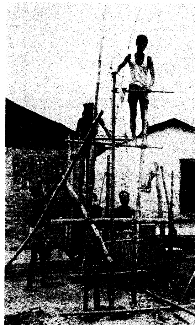
Figure 5.5 The palm-and-sludger method in use in Bangladesh (Photo: HEED, Dhaka Bangladesh)
