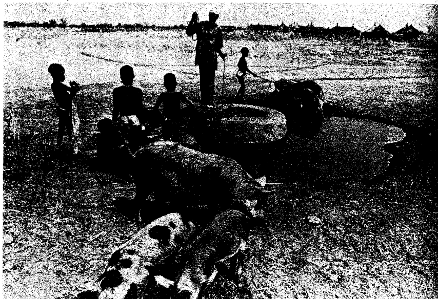
Figure 5.6 This well in Burkina Faso is contaminated by seepage of the pool of water around the well head into the well. The pool is contaminated by pig faeces (Photo: R. Witlin, World Bank)
